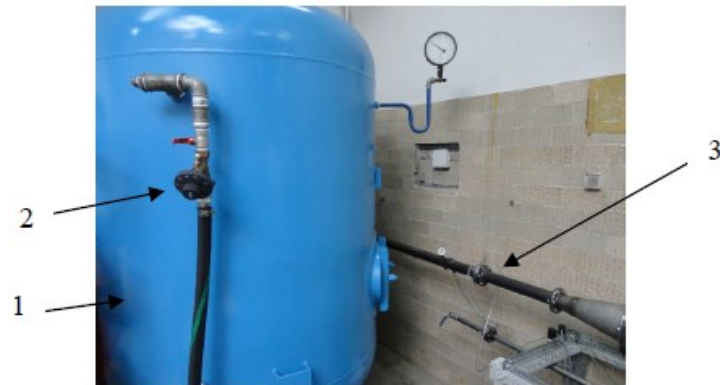
Fig. 2. The inlet part of the test stand: 1 – main cylinder, 2 – regulator valve, 3 – inlet channel
